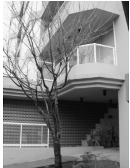
Look for trees growing close to balconies and windows that may act as a natural ladder.
